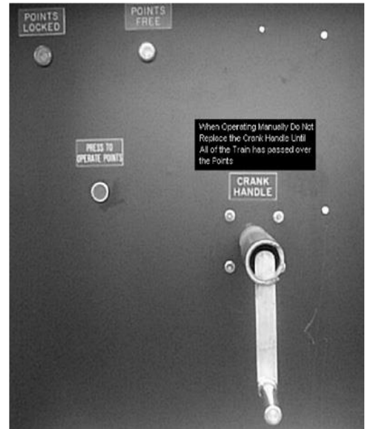
Figure 9022-3 Local control panel/crank handle case
