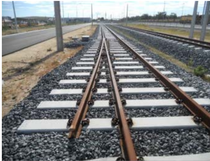
Figure 9012-9 Single Blade Catch Point.
