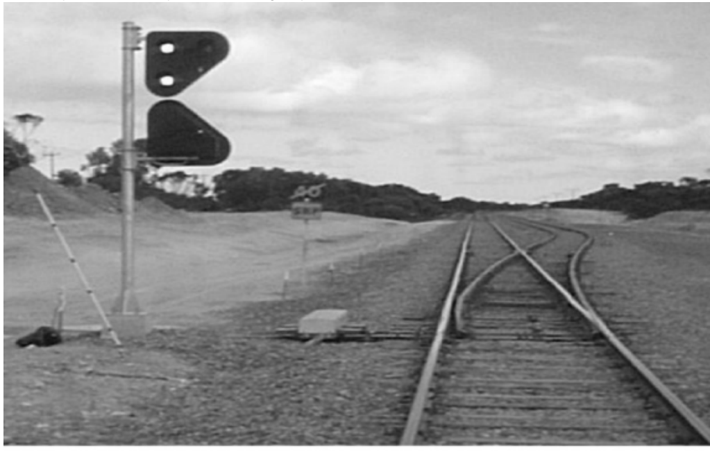
Figure 9022-1 Typical SRP Layout – white light type
