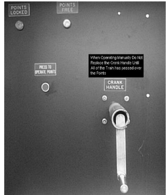
Figure 9022-3 Local control panel/crank handle case
