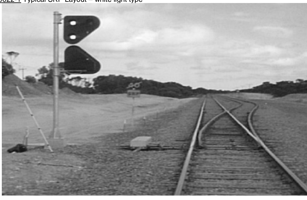
Figure 9022-1 Typical SRP Layout – white light type
