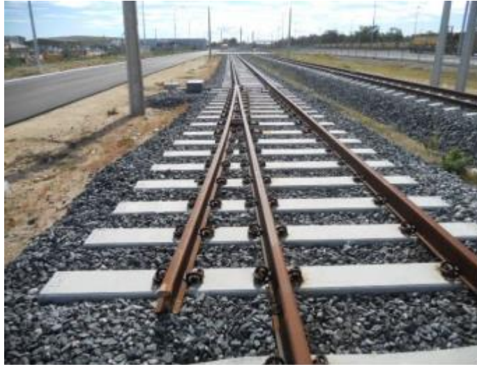
Figure 9012-9 Single Blade Catch Point.
