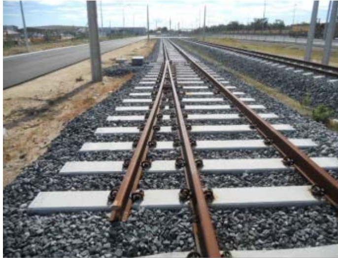
Figure 9012-9 Single Blade Catch Point .
