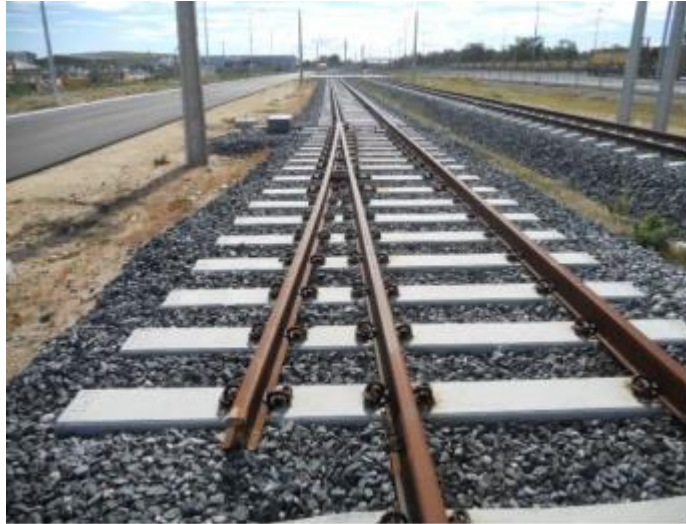
Figure 9012-9 Single Blade Catch Point.
