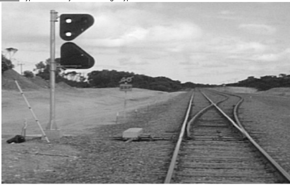
Figure 9022-1 Typical SRP Layout – white light type
