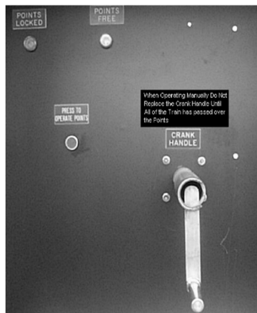
Figure 9022-3 Local control panel/crank handle case
