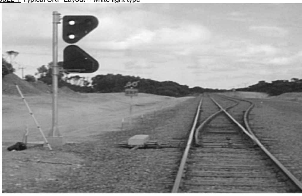
Figure 9022-1 Typical SRP Layout – white light type
