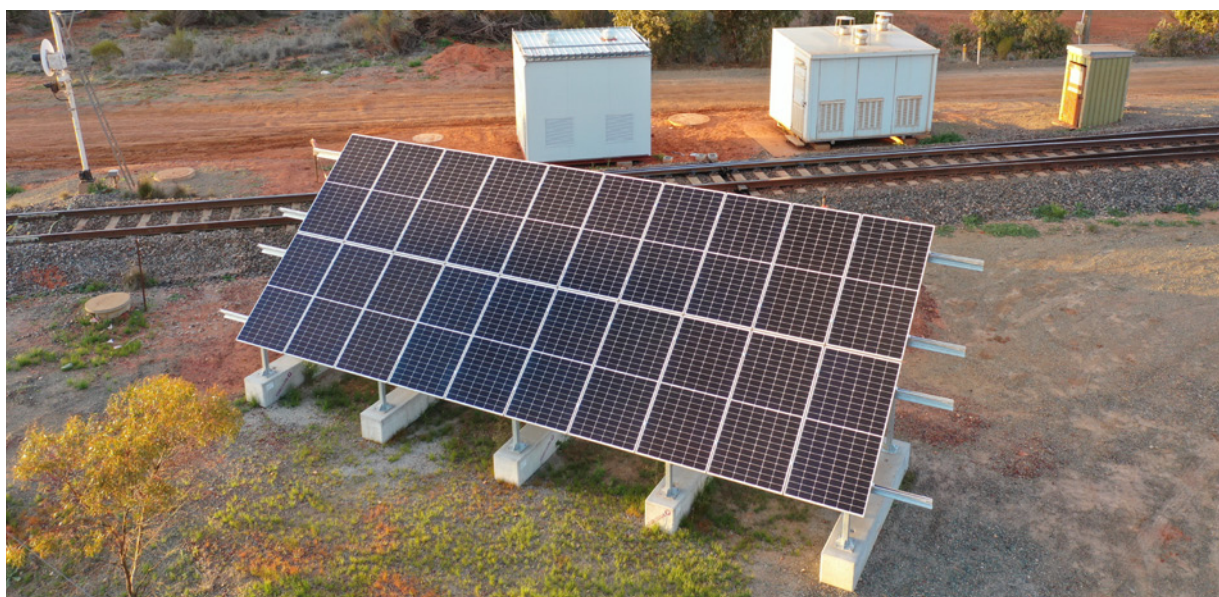
Off grid solar power supplies for signalling assets at Koolyanobbing.
