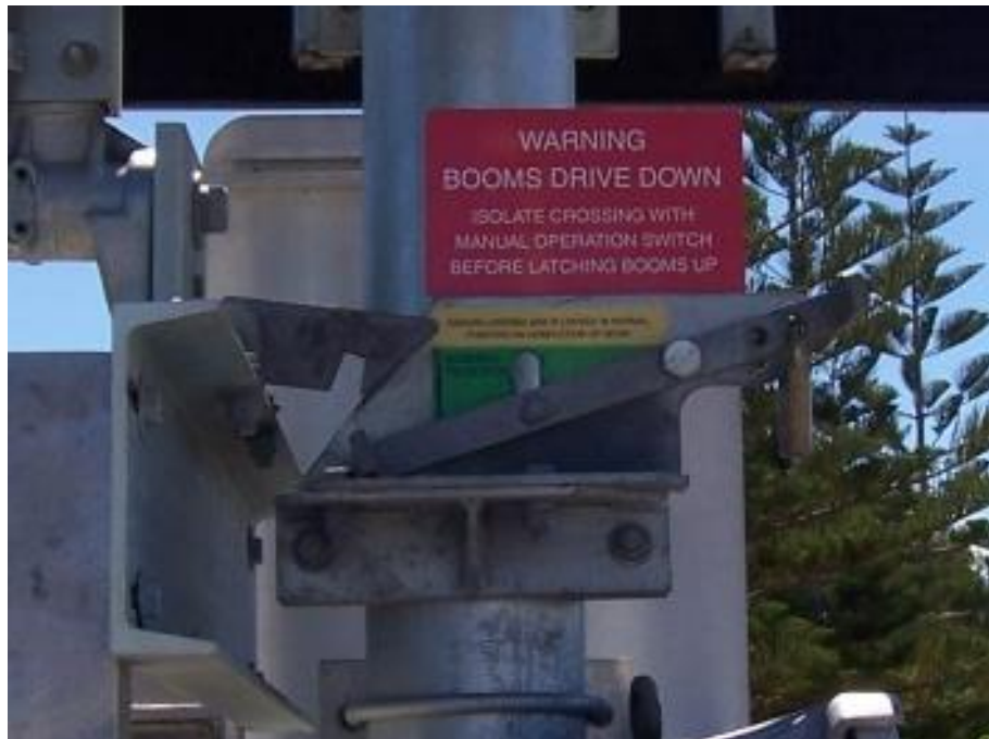
Figure 2015-1 Warning – Booms Drive Down sign.
